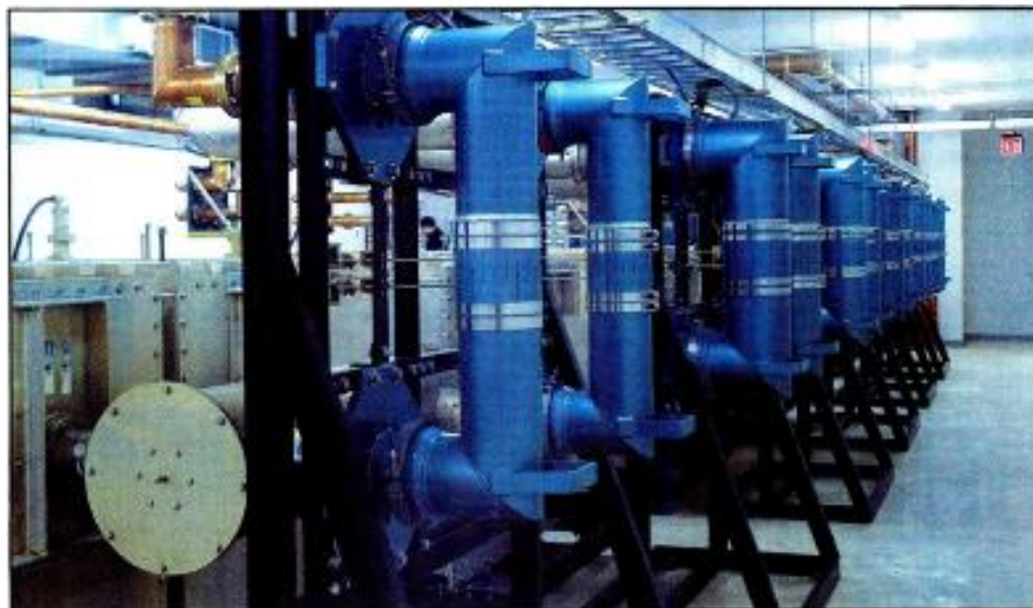
Multistation FM combiners have gained considerable interest since the FCC's 80-90 decision. Systems can be large or small, but the idea is always the same: Feed two or more transmitters into a single wideband antenna.
