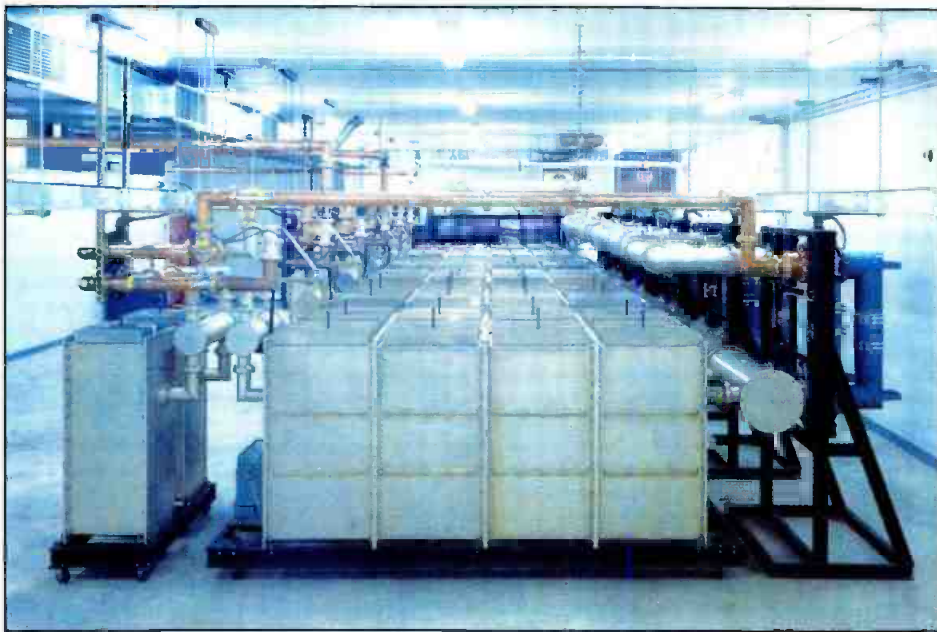
Large multiplexer systems require a great deal of floor space. Depending on the number of stations to be combined, the multiplexer may be configured to fit the physical space available. Note the use of casters on the individual modules of this combiner to make installation easier.
