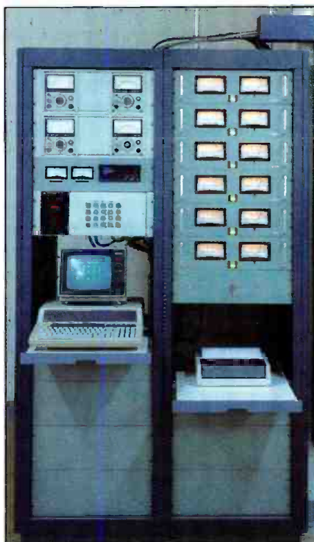
Accurate and complete monitoring is essential to a reliable multiplexer system. The arrangement shown features continuous monitoring of forward and reflected power for each of the six stations using the multiplexer. A computer processes electrical and environmental data to manage site operations.
